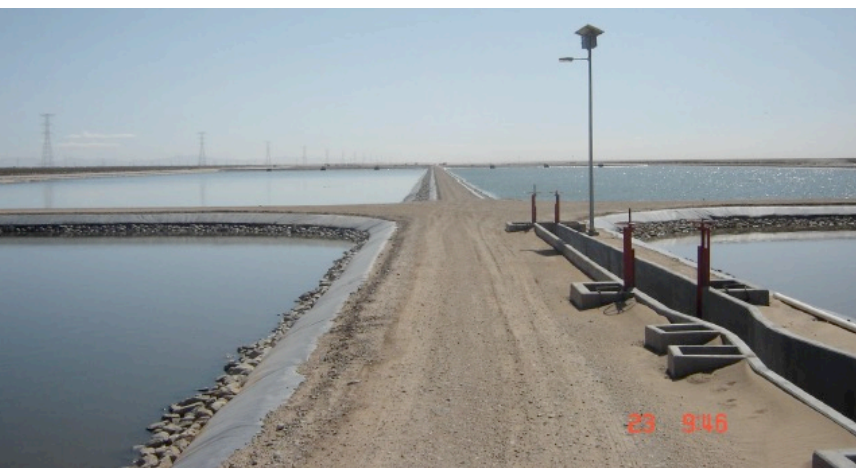
Operational infiltration basins of 0.014 km 2 each. Total infrastructure cost of approximately USD 660,000 (photo: H. Hernandez).
