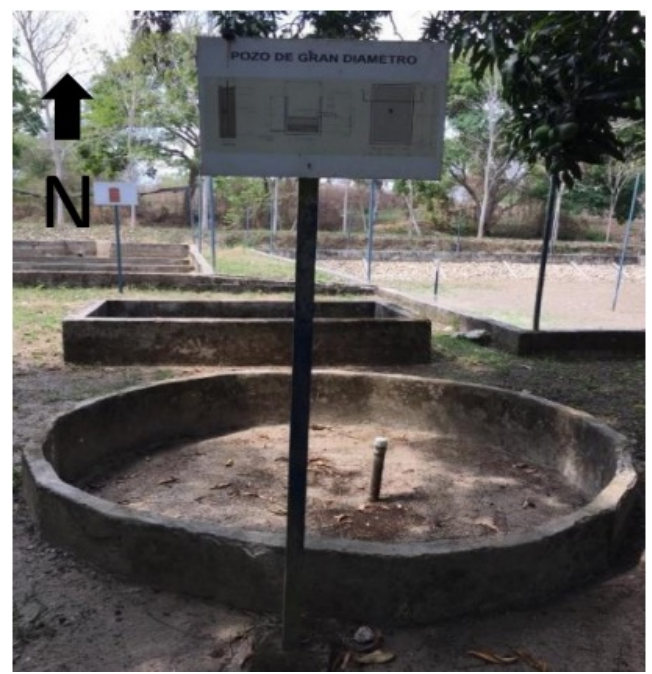
Large diameter well (photo: José Luis Navarro, 2020).
