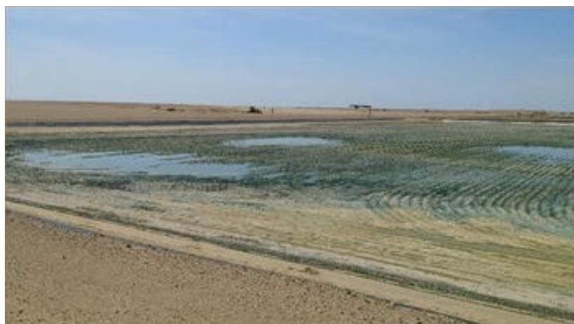
Clogging of infiltration pond soil, causing reduced infiltration and loss of surface smoothness (photo: Humberto et al., 2018).
