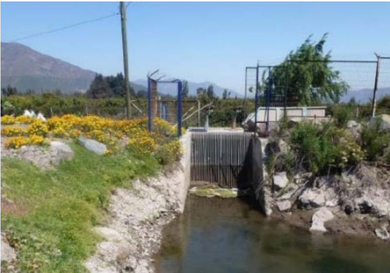
Surface intake diverting water from the Aconcagua river towards Las Vegas water treatment plant (photo: SISS, 2014).
