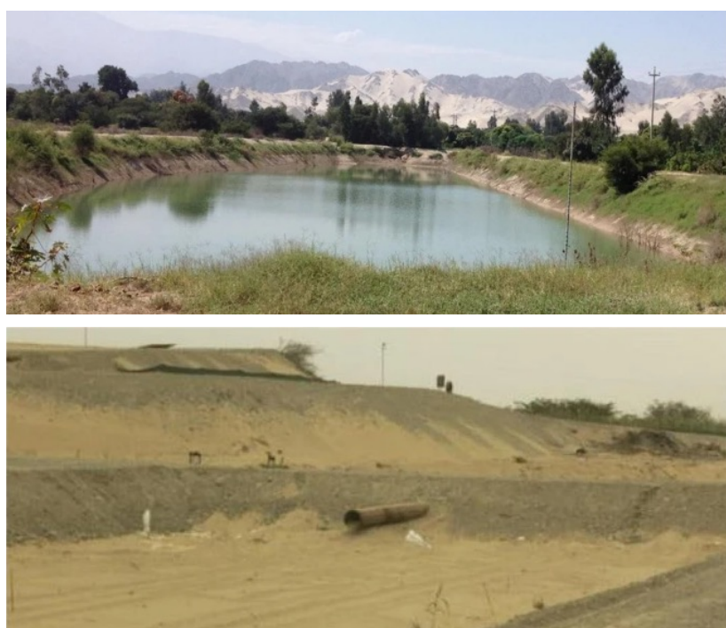
Full (top) and empty (bottom) infiltration ponds (photo: Enrique Fernández-Escalante).
